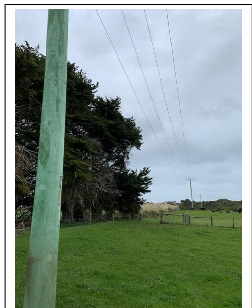
Location 4 Pole 209 (Cypress 3.5 Metres – Code 2024
